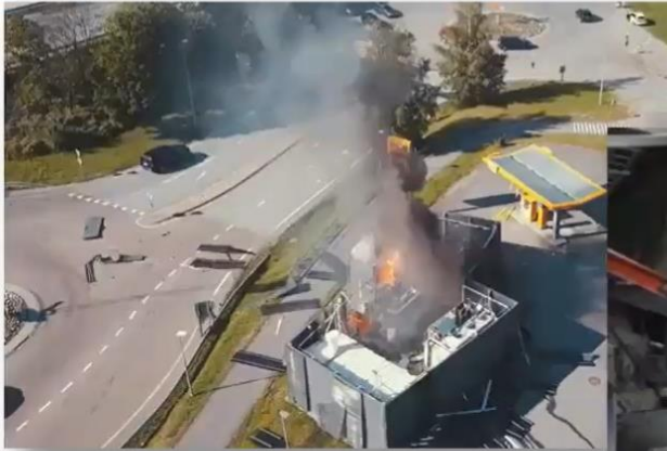
Norway, 2019 Hydrogen fuelling station explosion
