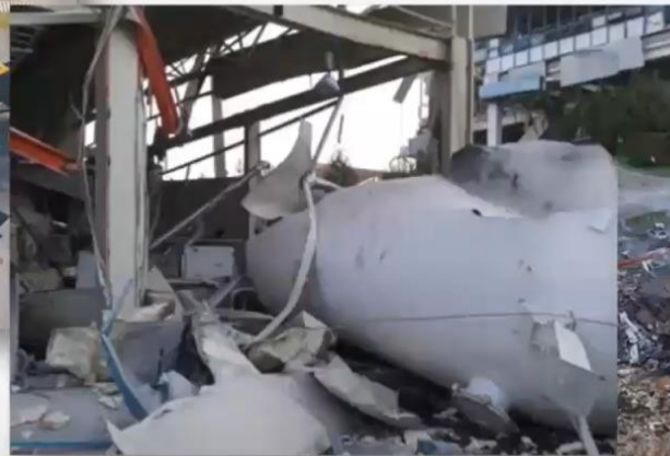
South Korea, 2019 Hydrogen tank explosion
