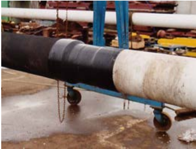
COMPLETED HEAT-SHRINK SLEEVE OVER A GIRTH WELD
