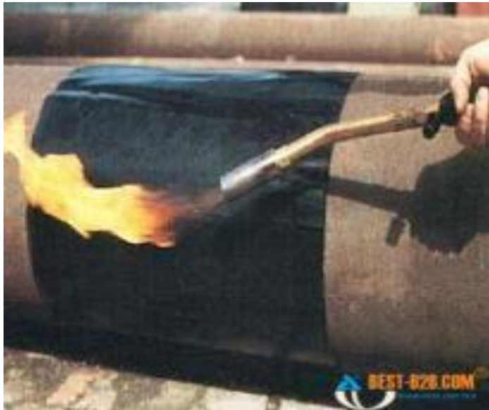
APPLYING A HEAT-SHRINK SLEEVE
